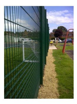
Fencing is usually erected to 3.0m with 4.5m behind goals and in areas where containment of balls is important e.g. adjacent to roads. It typically comprises weld-mesh panels suspended from box section posts. Close gauge mesh can be used in goal areas and other areas of high impact for better resistance.
